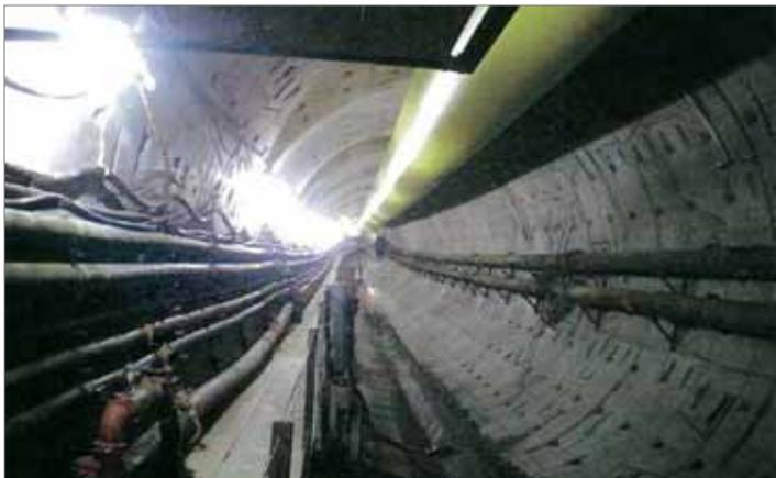
**Figure E-11. Typical TBM Tunnel during Construction**
